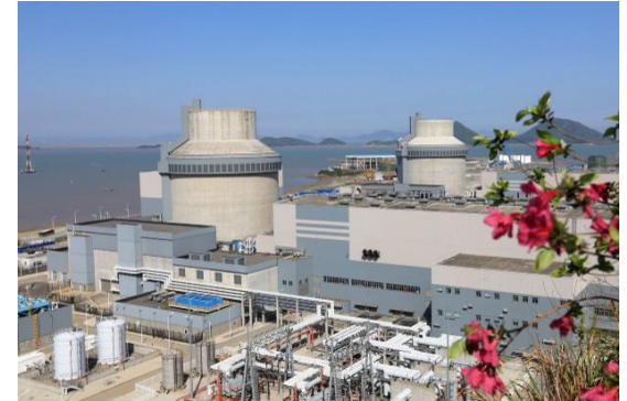
AP-1000 (Westinghouse) in Sanmen (CN), 1200 MW
