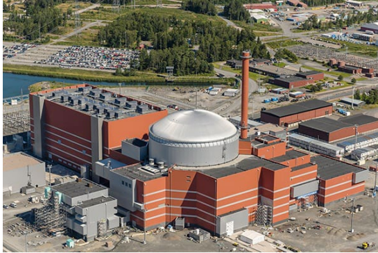
EPR (Framatome) in Olkiluoto (FI), 1600 MW)
