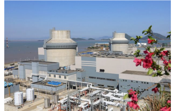
AP-1000 (Westinghouse) in Sanmen (CN), 1200 MW
