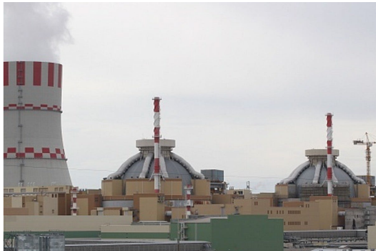
VVER-1200 (Rosatom) in Novovoronezh (RU), 1250 MW
