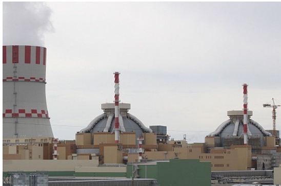
VVER-1200 (Rosatom) in Novovoronezh (RU), 1250 MW
